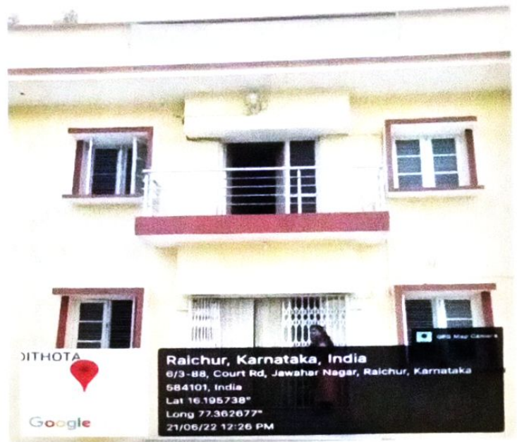
Hostel Entrance Camera
